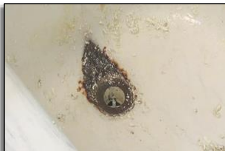
Erosion damage & rust under the drain
