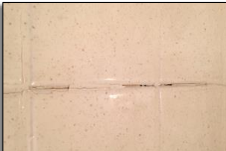
Grout problems where not addressed before refinishing
