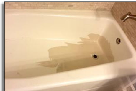
Failed refinishing requires chemical stripping
