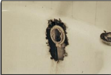
Overflow - drain rust out
