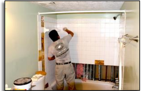
Tile repair wet wall damage
