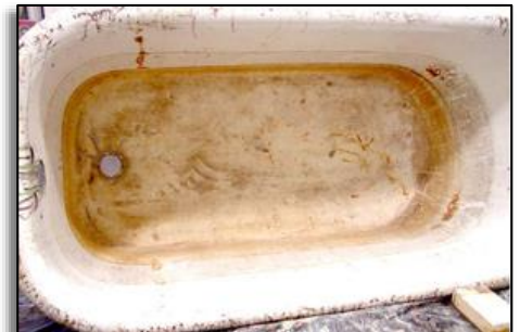
Clawfoot tubs often require extra repair work in the bottom and suffer rail damage.
