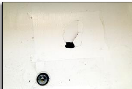
Cracked hole fiberglass tub
