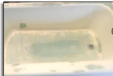
Heavily damaged bottom & rail rebuild
