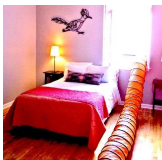
Exhaust To A Window Away From The Bathroom
